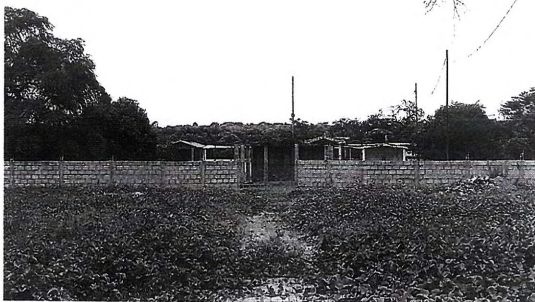
CEMENTERIO CAPILLA CENTRAL
