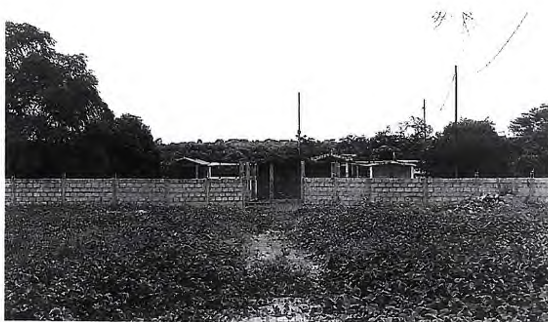
CEMENTERIO CAPILLA CENTRAL
