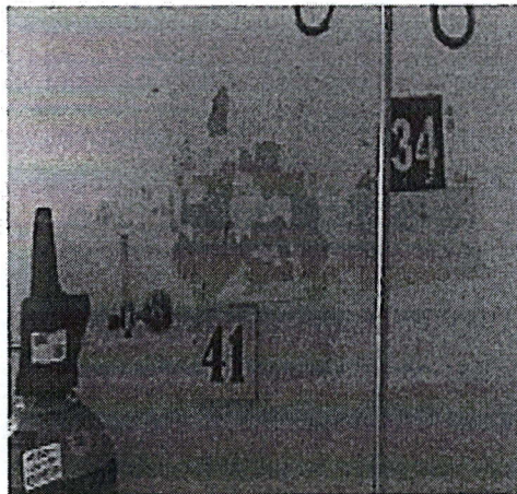
Paredes salitrosas - Hospital II Cañete EsSalud
